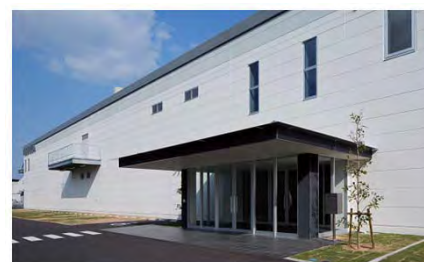
External view of new office building
