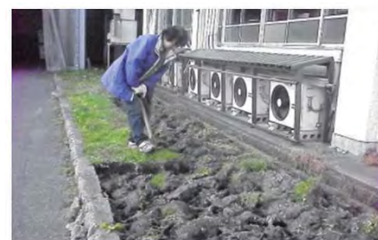
Work to replace the soil
