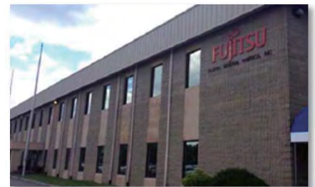
Office building of FGAJ
